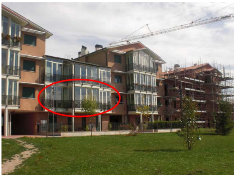
Figure 5. View of the south-west façade of the building, with the flat used as case study.
