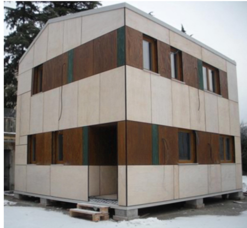
Fig. 1. The test building of the University of Trento.
